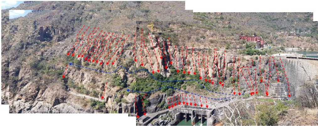
Figure 3. Inspection paths used during the geotechnical survey
